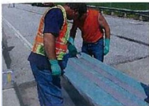
(c) Epoxy application on laminates
