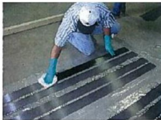
(b) Cleaning CFRP laminates
